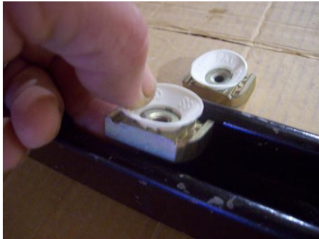
Insert a strut nut into channel.
